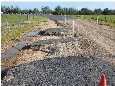
Again. When Leighton Contractors decided to use sand as the road-base when upgrading Geregarrow Road, why wasn't that questioned by one of councils many engineers? That could have prevented the bitumen from 'floating' off the sand with every flood. Where the most recent flood, February 2022, washed the bitumen off yet again, no warning signs have been erected, and 3 months on, nothing has been done to fix it.
